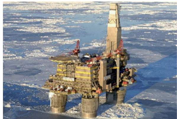
Fig. 7. Ferro-concrete ice-resistant stationary platform in the Sea of Okhotsk
