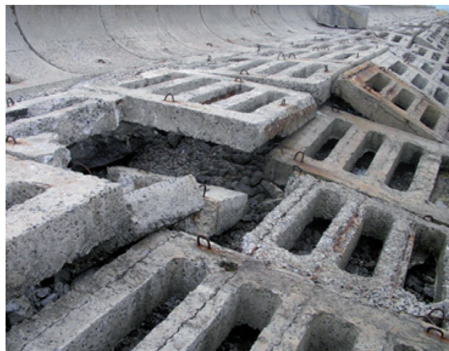
Fig. 1. The current technical condition of the coastal protection structures of the passive type on the Odessa coast (B. Fontansky cape)
