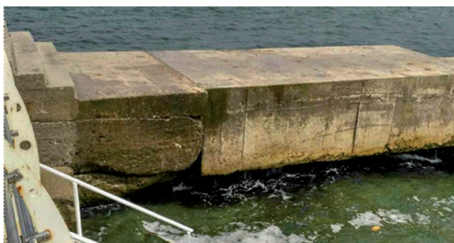
Fig. 2. The state of the root part of the buna in the zone of the variable water horizon
