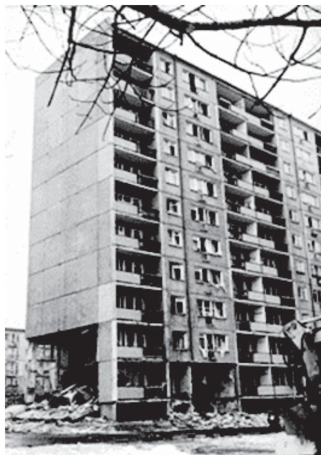
Figure 6 - Effects of a gas explosion in a large-panel building (Łódź, Retkinia housing estate)
