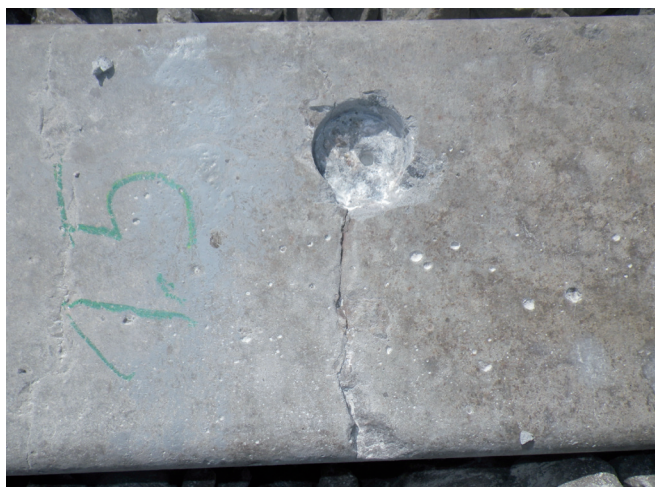
Figure 5 – Cracks within concrete sleeper
