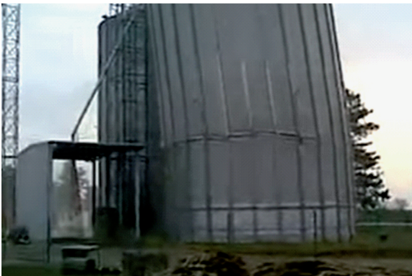
Figure 3 - Segment of video recording the silo deformation and destruction beginning
