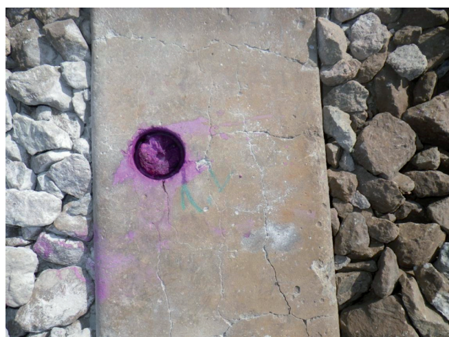
Figure 8 – Cracking on the sleeper produced in 2010
