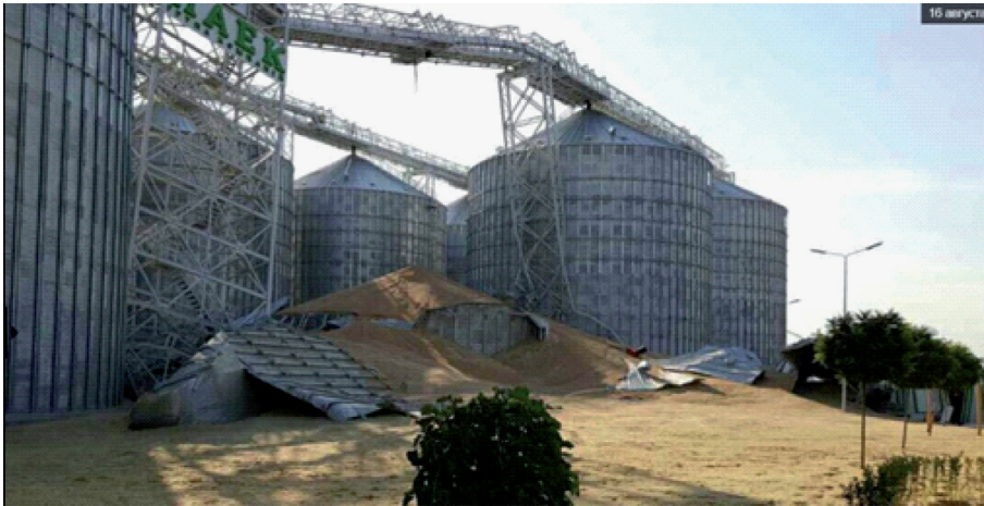
Figure 2 - Grain silo destruction consequences
