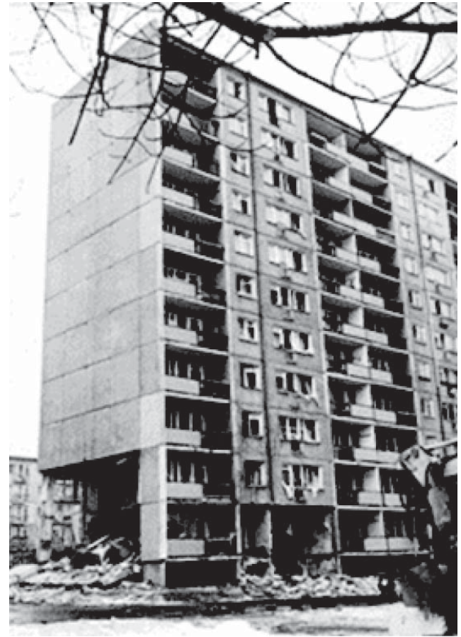
Figure 6 - Effects of a gas explosion in a large-panel building (Łódź, Retkinia housing estate)
