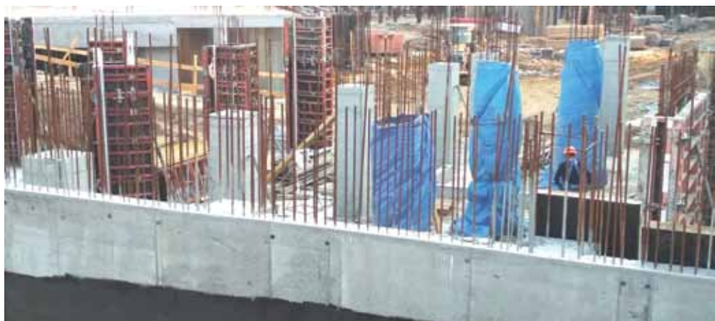
Figure 1 - General view of the formed vertical structures
