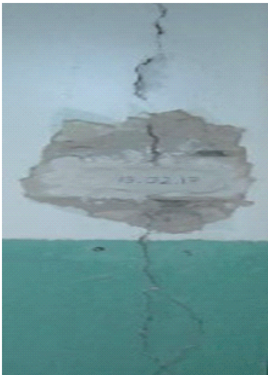
Figure 2 - Chalky screed after the installation of the pile
