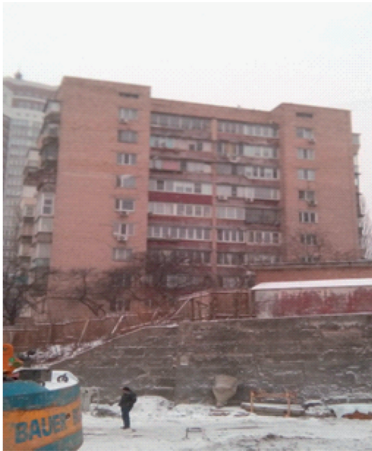
Figure 1 - Investigated building and retaining wall - View
